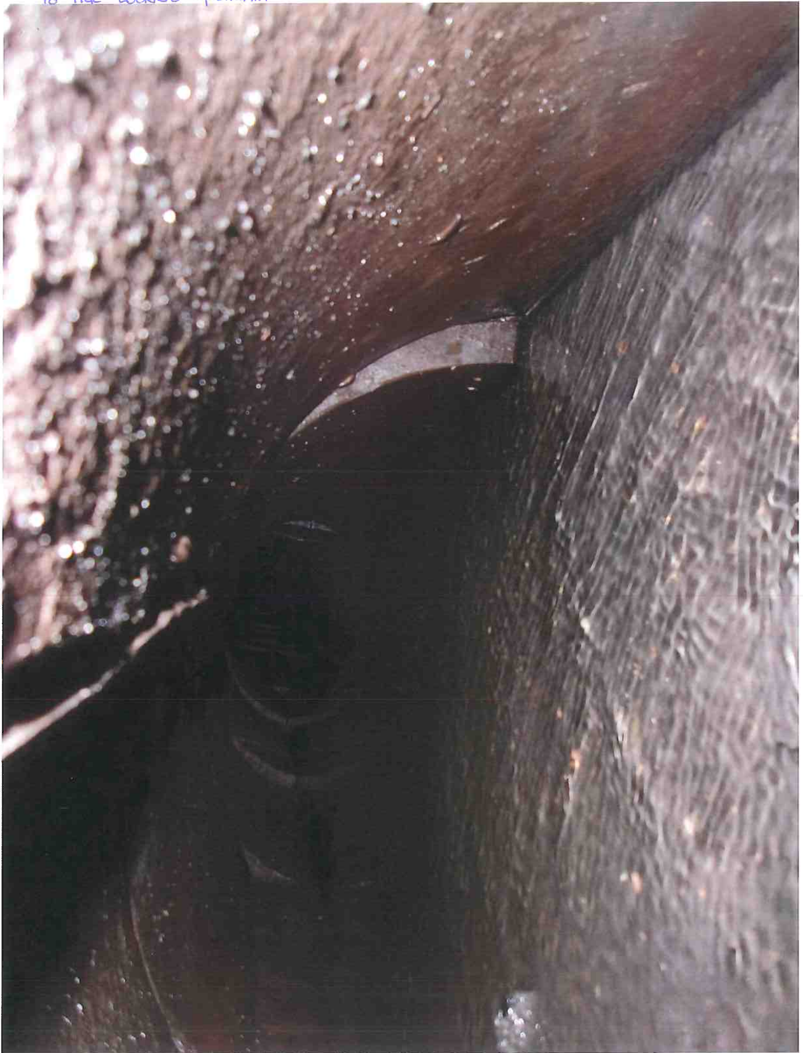
18" TIE Looking Upstream
